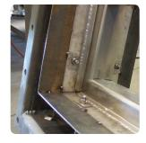
Because there are no seal cavities, there is no area to collect ash and sludge deposits, and corrosion attack of the metallic seals is mitigated.
