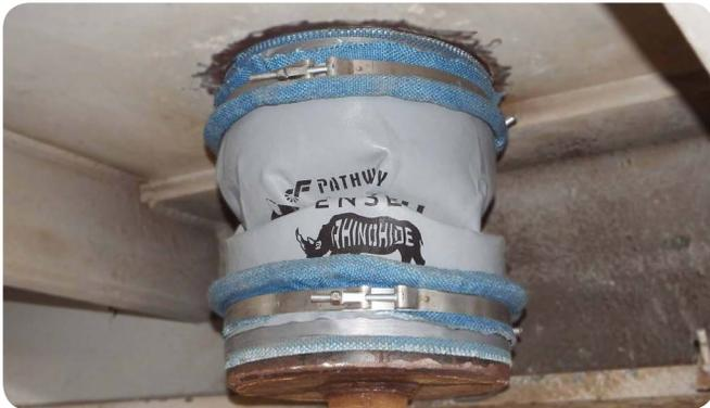
Penetration seals may be exposed to high cycling frequency. They may be exposed to high temperatures, up to 1150 Fahrenheit in some cases. Tight Clearances between multiple penetration seals and also between penetration seals and existing support structural steel.
